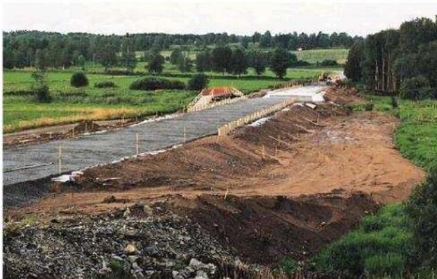
Figure 3.6 LLP-Light loadspreading plate
