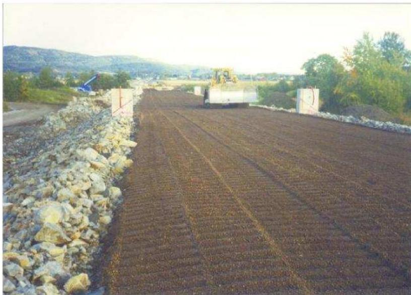
Figure 3.4 LWA as frost insulation in railroad embankment, Vestfoldbanen, Norway
