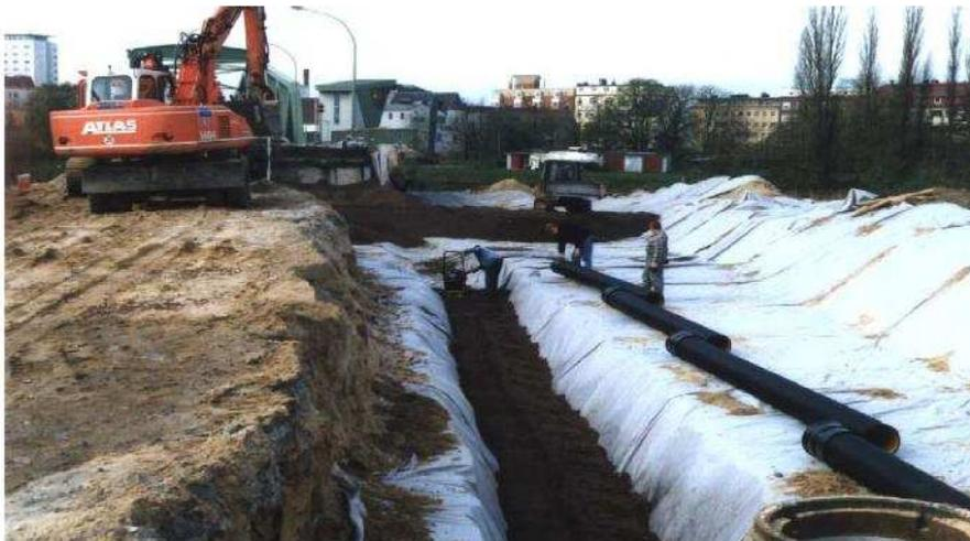
*Figure 5.4 LWA in drainage ditch*
